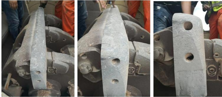
MIMC -Cr2021 板锤安装 MIMC -Cr2021 blow bar install
